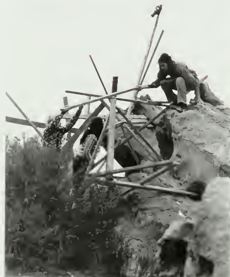
178 Making structures of 2 x 4s
