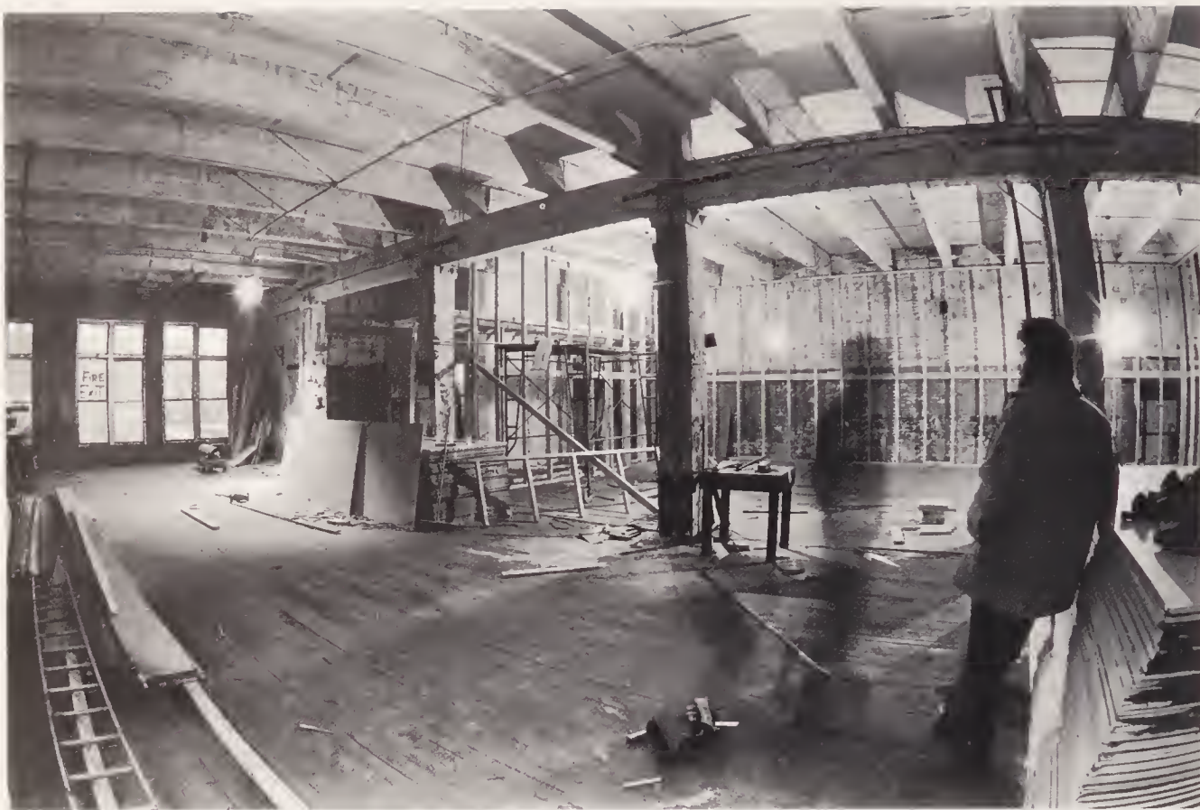
8 Construction photograph, Amba and Razor , 1982
