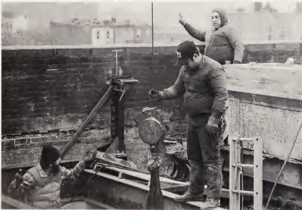
21 Construction photograph, Meeting , 1980
