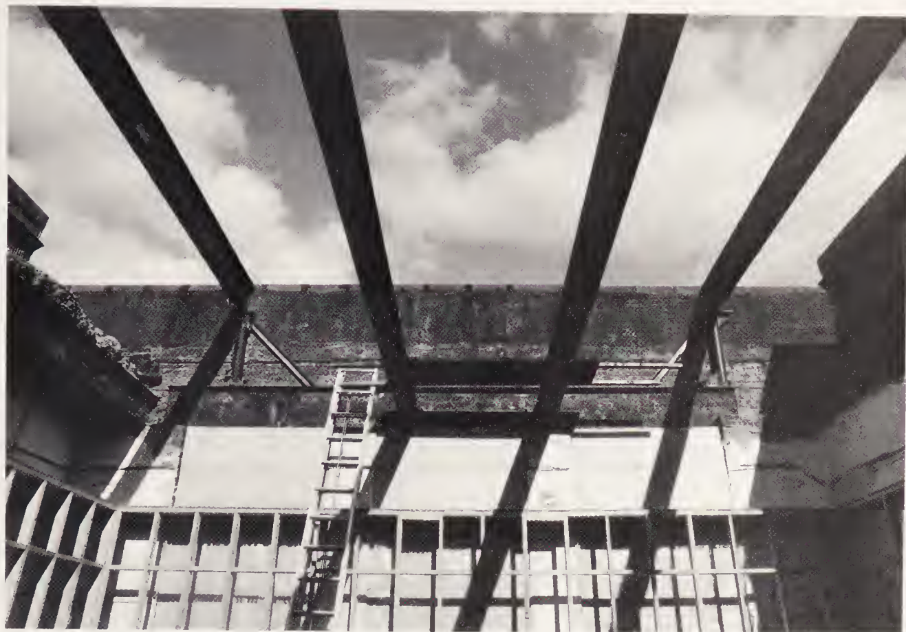
22 Construction photograph, Meeting , 1980
