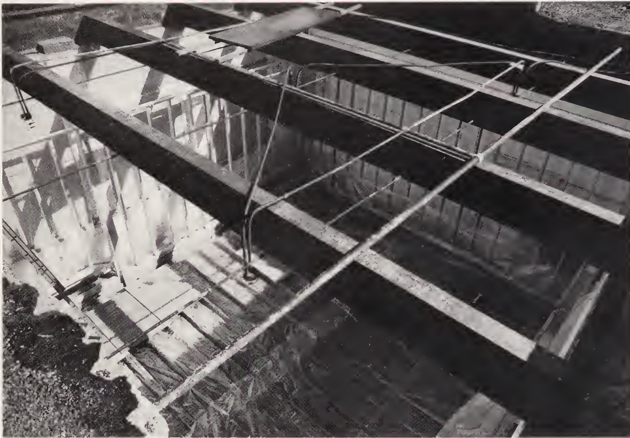
20 Construction photograph, Meeting , 1980
