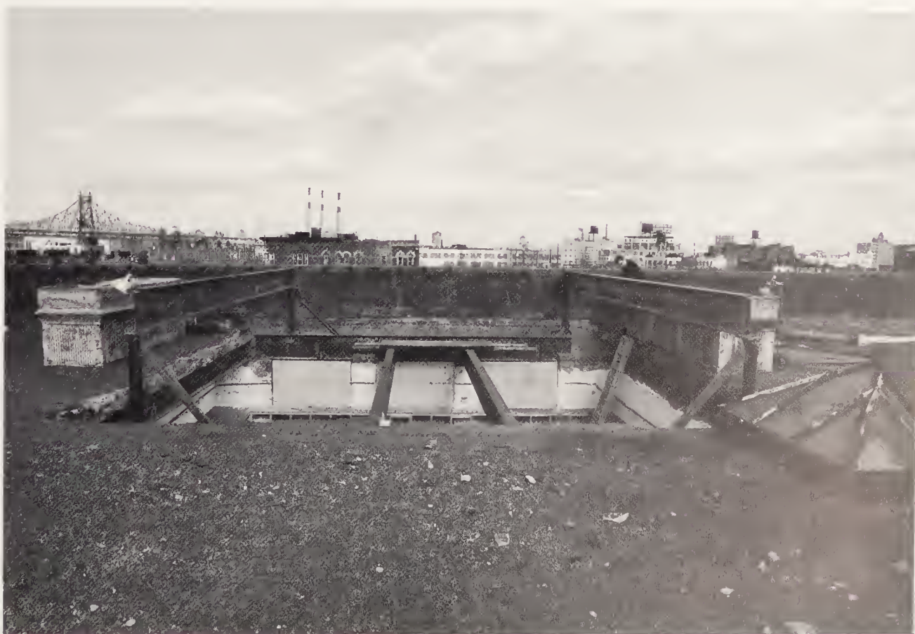
23 Construction photograph, Meeting , 1980
