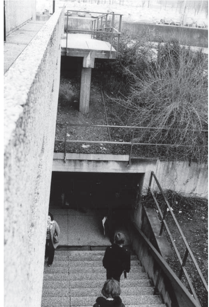
FIGURE 2.3 Pedestrian Underpass, Münster
