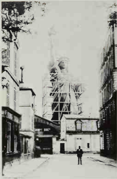
Swathed in scaffolding and towering above the narrow Paris streets, the Statue of Liberty nears completion in the outdoor studio of sculptor Frédéric Auguste Bartholdi, who worked on the 151-foot figure for 10 years. Commissioned by a sympathetic group of French citizens as a gesture of friendship to the United States, the statue, whose proper title is "Liberty Enlightening the World," was taken apart and shipped to New York. There it was erected on an island in the harbor and formally dedicated in 1886.
