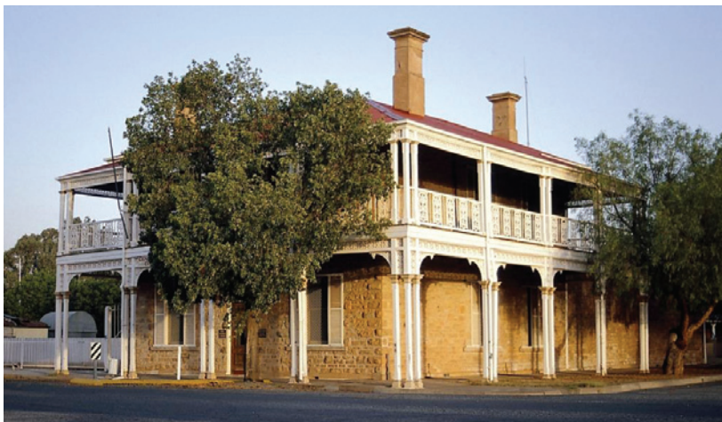
Figure 5 Central Darling Shire chambers on Reid Street, 2003 (built 1890).
