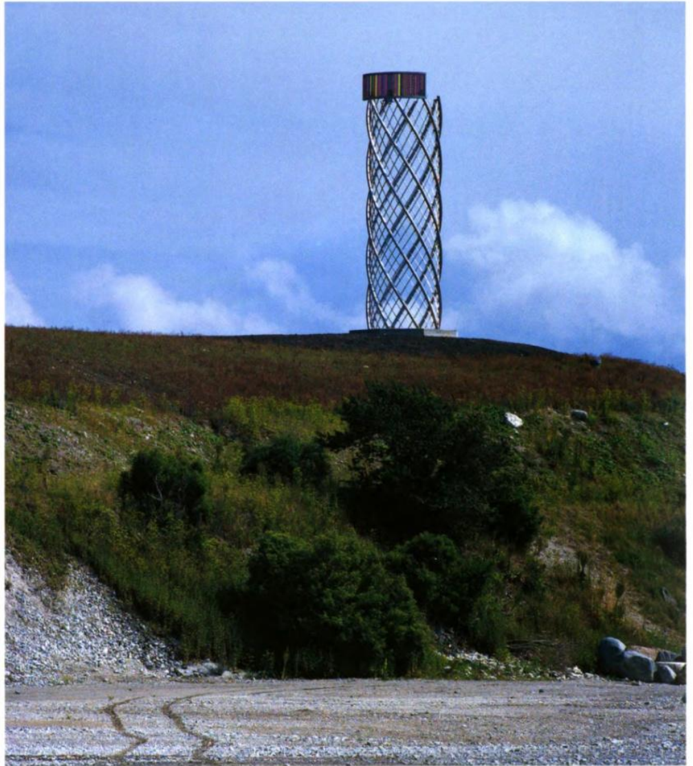
The movement meter tower for Lernacken 2000 Steel, light, colour spectrum h. 12.63 m, ø 4 m Installation, Malmö, Sweden Collection, City of Malmö, Sweden
