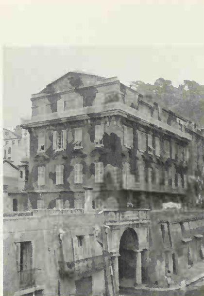
Matisse occupied a balconied top-story apartment in this building in Nice for 17 years. Although he fled the Côte d'Azur's burning, blinding sun in the summer, the apartment remained his home base from 1921 to 1938. The photograph above, taken during World War II, shows the yellow-washed building splattered with dark paint for camouflage against air raids.
